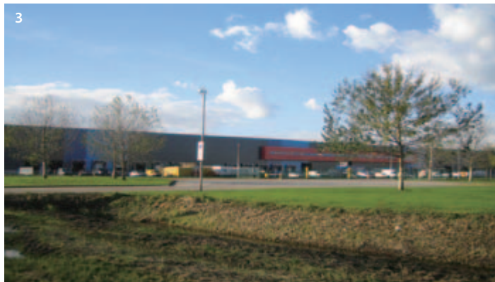
* 1. Warehouse facility 2/3. Recently completed Moerdijk distribution facility
